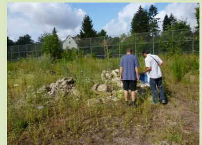
Brownfield with concrete leftovers
