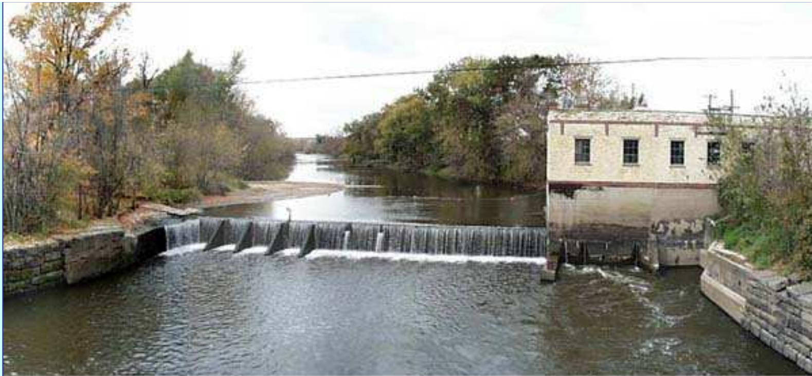
Linen Mill Dam, Baraboo River (above). Removed October, 2001 (below).
