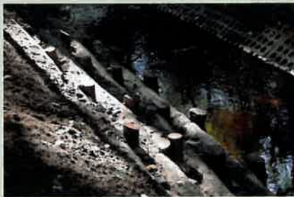
Stream bank of Ślepiotka: concrete blocks replaced by wooden elements, August 2010
