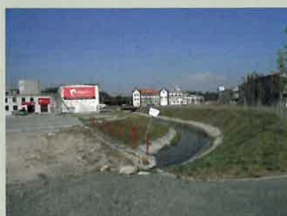
Area at former Brno Škrobárny factory selected for revitalisation
